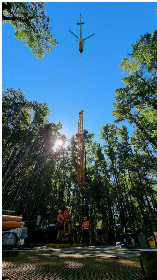
Figure 1. CS1500 mast being flown into Alexander River.
